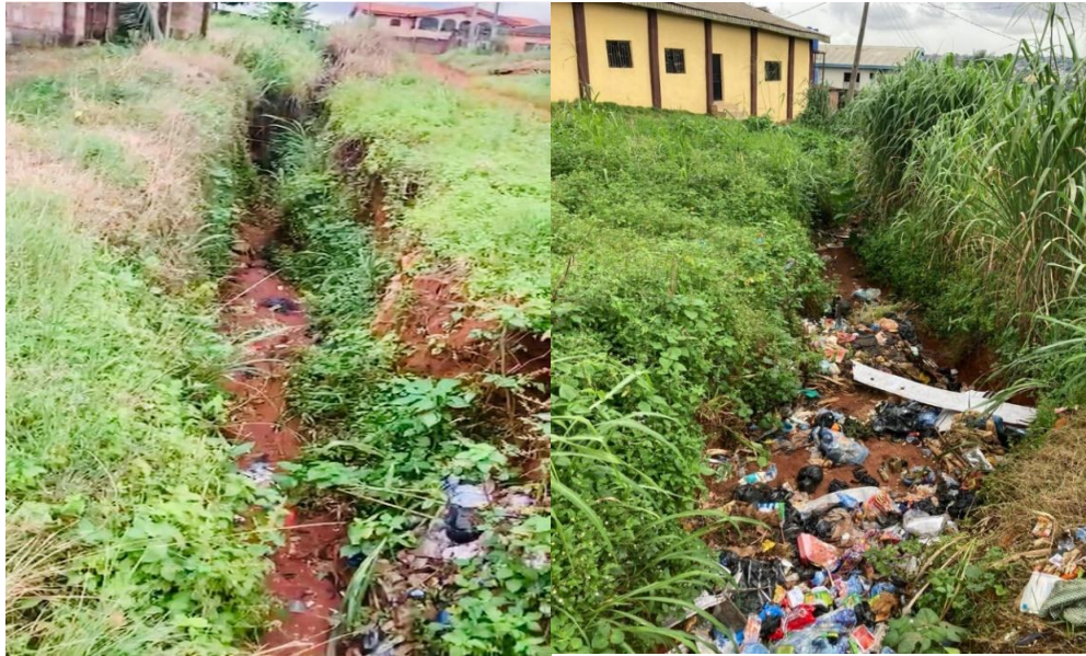
Fig. 2(c)View of gully erosion in the study catchment Fig. 2(d)Gully scar used as waste dumpsite
